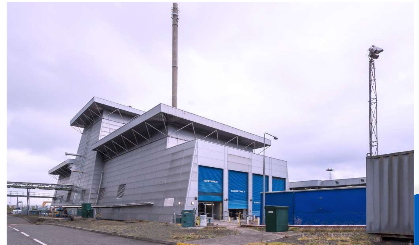
Mono sewage sludge incineration, Belfast, Northern Ireland Capacity: 24,000 t/a (sewage sludge, dewatered sewage sludge, screenings from the the sewage treatment plant) Multi-stage flue gas cleaning system incl. electrostatic precipitator
