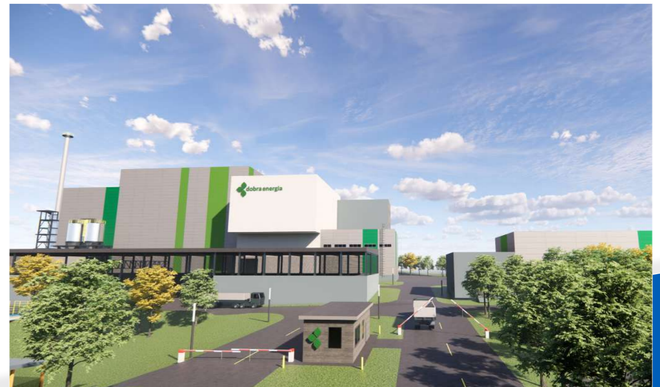
Thermal waste treatment, Olsztyn, Poland Capacity: 1 x 110,000 t/a (RDF) Gas volume flow: 1 x 92,000 m 3 /h (STP, wet) Circoclean® flue gas cleaning
