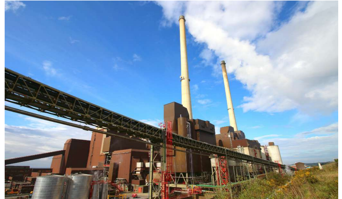
The SCR system installed at the Moneypoint plant in Ireland is operated with urea as a reducing agent
