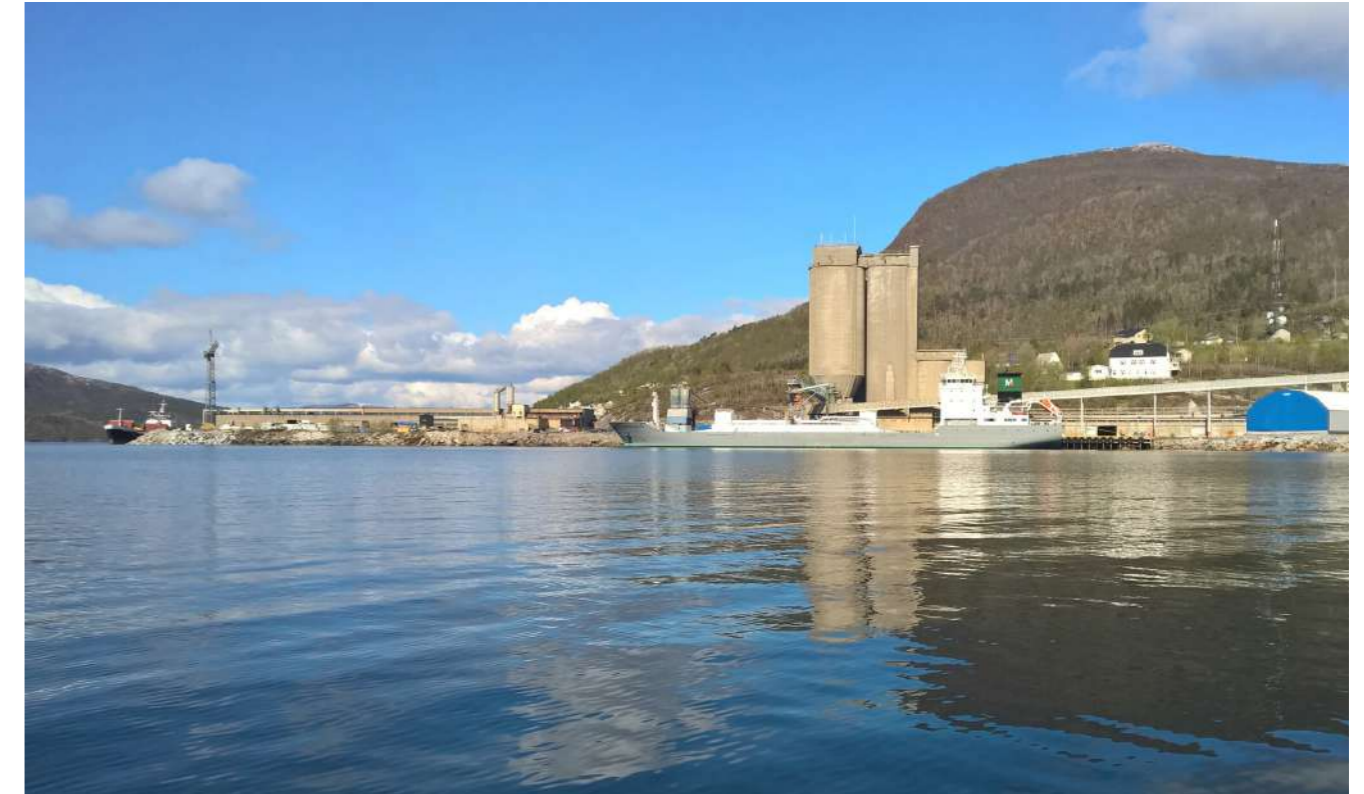
Cement plant, Kjøpsvik, Norway Gas volume flow: 280,000 m 3 /h (STP, wet) Alkaline wet scrubber
